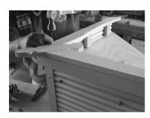
STEP 5 Cut the barge caps (L) with a 45° angle at each end and screw through the roof to the battens, making sure they are flush with batten ends. Use the gridded diagram
