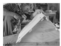
STEP 4 Cut the roofing (J) to size and screw to the battens at about 200 to 250mm spacings along the roof. Predrill through the tops of the corrugations and use roofing screws with a neoprene seal to keep the roof watertight. Add the ridge cap (K) to cover the top roofing join.
