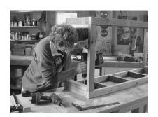
STEP 2 Build the floor and top frames by screwing the long rails (C) to the short rails (D). Screw **Continued overleaf**
